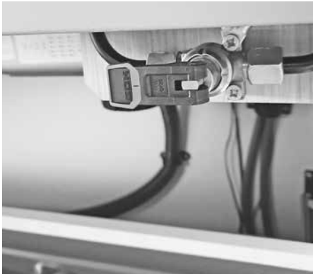
Shut-off valve in the kitchen
